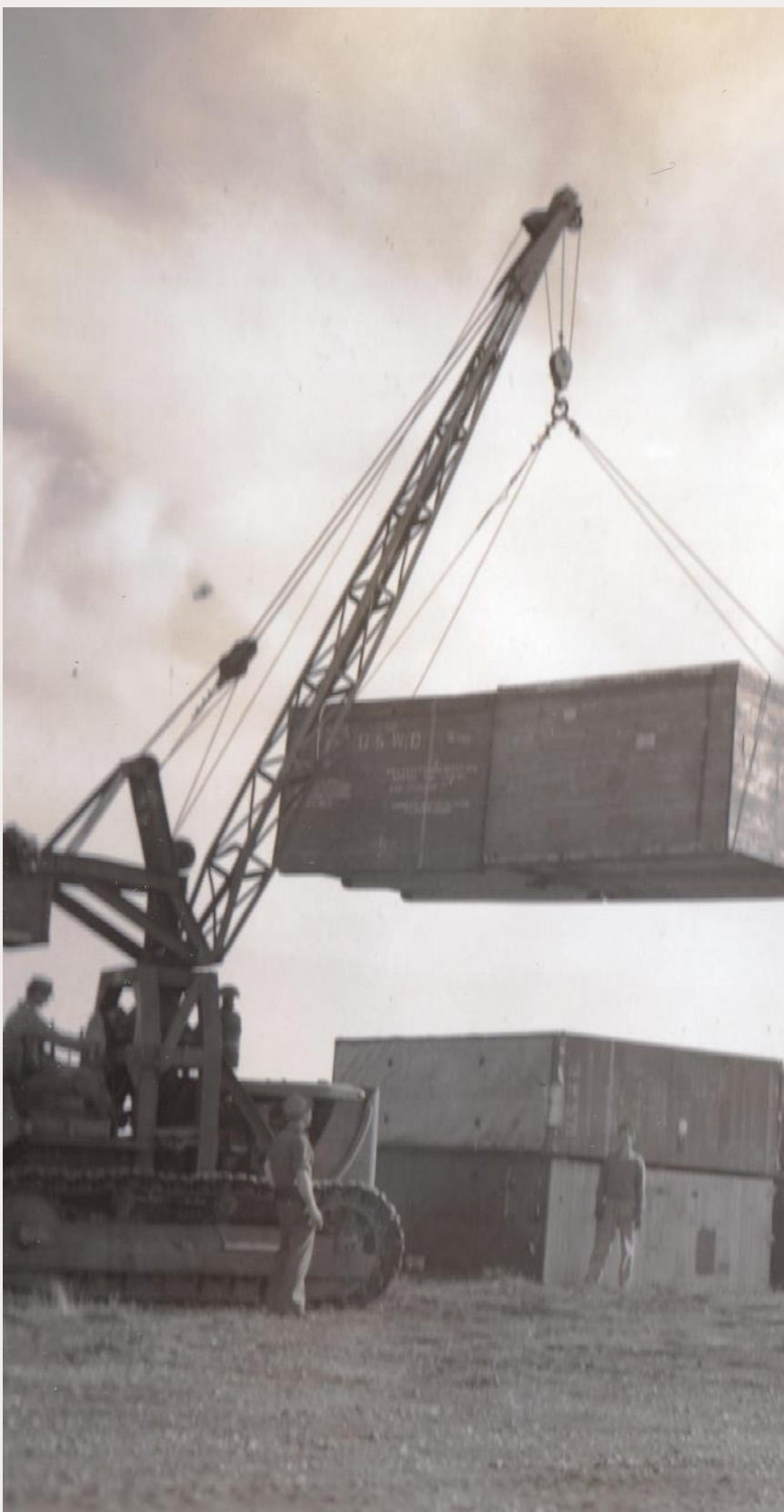
Crane lifting crates with glider parts. This photograph is probably taken at Greenham Common where many of the gliders for the ETO air lifts occurred. It does show how the crates were moved from ships or trains. (Photo Courtesy of National Archives, USAAF photograph)
