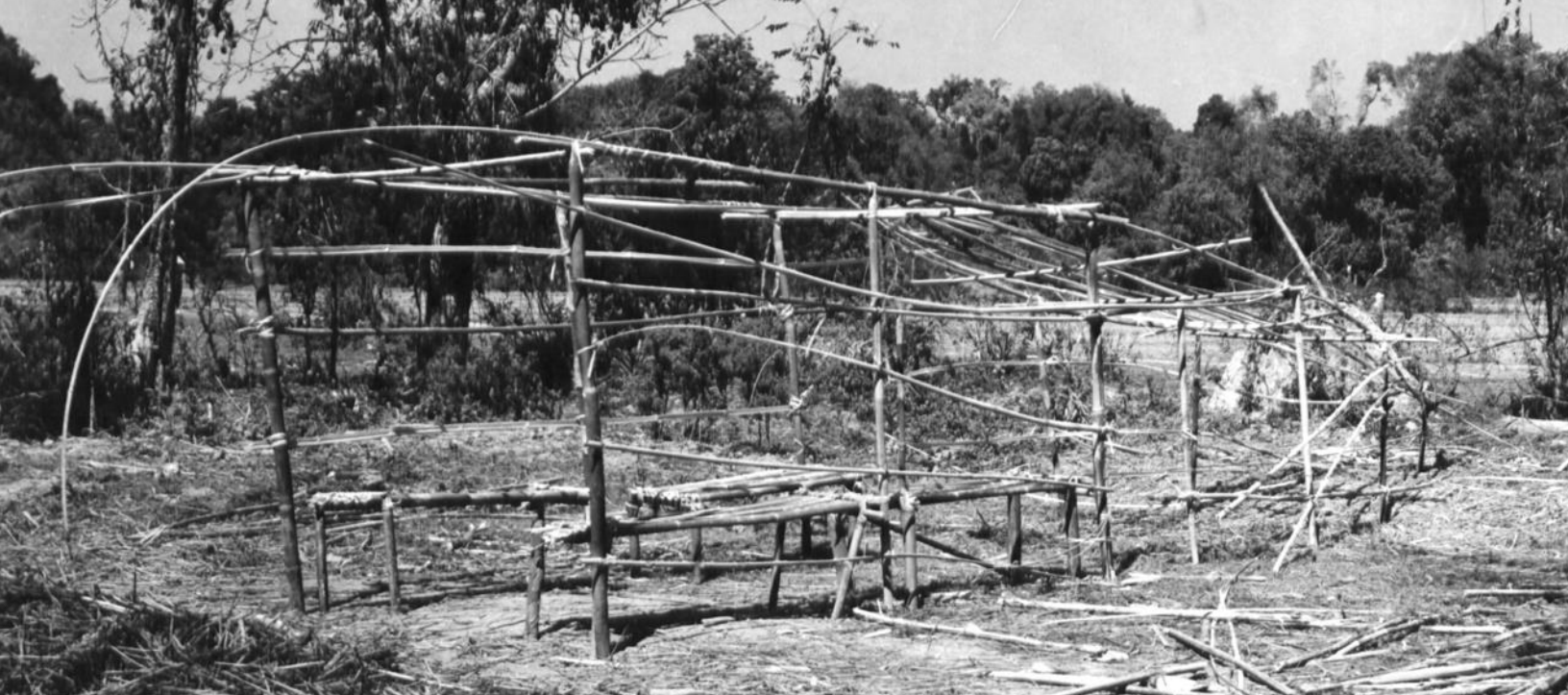
Glider mock-up built of bamboo for practice seating of "Gurka" troops of the 1st Air Commando Force based at Hailakandi, Assam, India. The CG-4A glider specification for seating was 15. Two pilots and 13 troops. It was documented that the gliders were loaded with 16 to 18 Gurkas. And over weighted with unauthorized extra ammunition.
