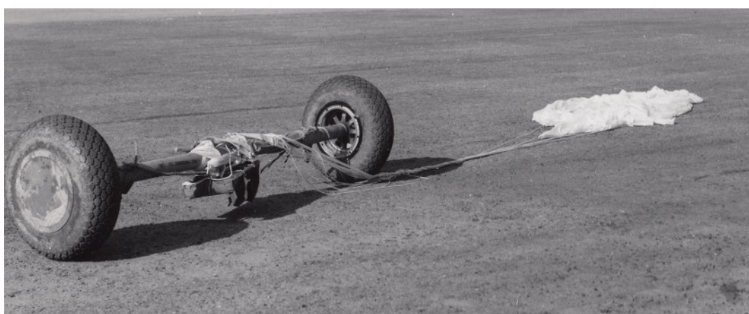
Caption: The landing gear, dropped by a glider participating in the 52nd troop Carrier Wing Maneuvers in 1943, [the gear] landed on Comiso Air Field Sicily. Both the gear and the parachute are in good condition. Photo Source: U.S. National Archives, courtesy of the NWWIIGPA research team.
