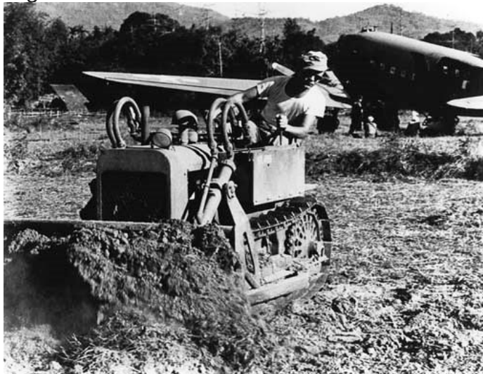
Invasion of Burma at landing zone Broadway. Gliders brought in three bulldozers; within 24 hours, airborne engineers had prepared a landing strip 300 feet by 5,000, ready for use by more gliders and Troop Carrier Command C-47s, bringing in more men, animals and supplies. NARA posted on Olive-drab.com
